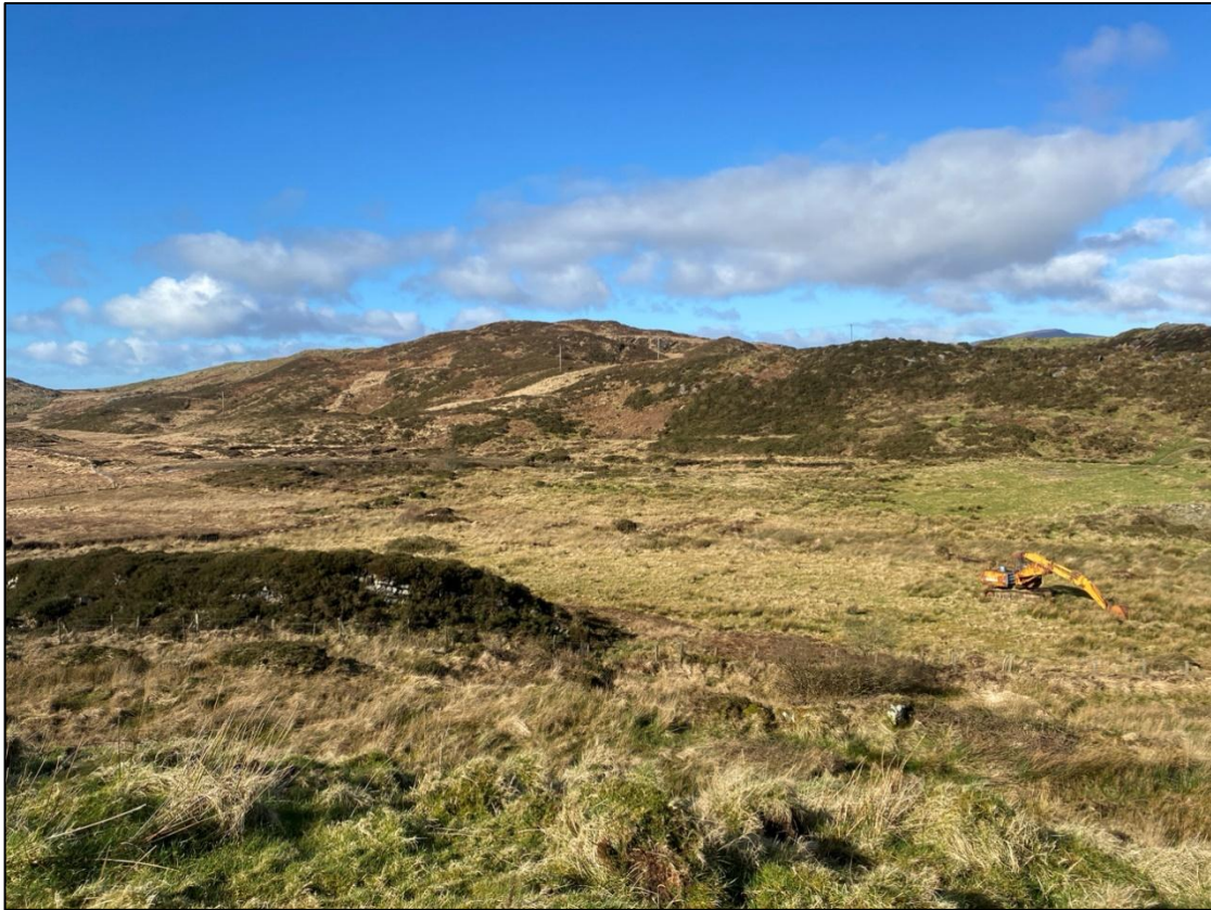
Plate 3-22 Access Road linking T12 to T13, located on undulating Wet Grassland (GS4)/Scrub (WS1) in the west of the Proposed Wind Farm southern turbine cluster.
